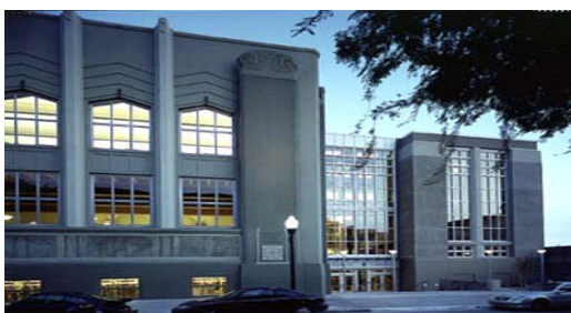
Berkeley Central Library
